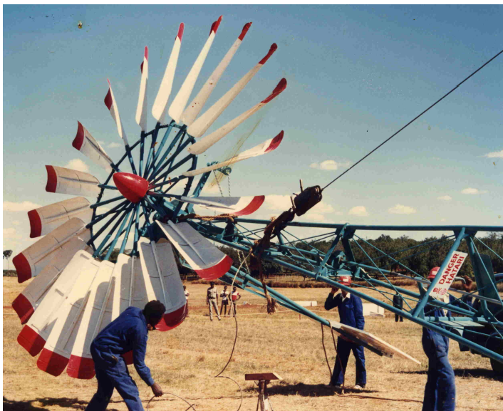
Above: Our Kijito towers are hinged so they can be assembled at ground level and then winched into position. Below: Pumping water for elephants in Tsavo Park
